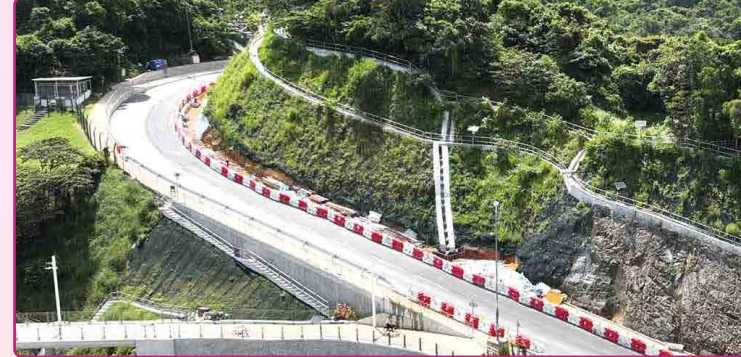
東涌道北的道路擴闊工程已大致完成 Road widening works at Tung Chung Road North were substantially completed
