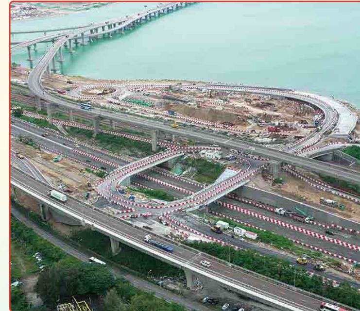
大蠔交匯處的道路及渠務工程 Road works and drainage works for Tai Ho Interchange
