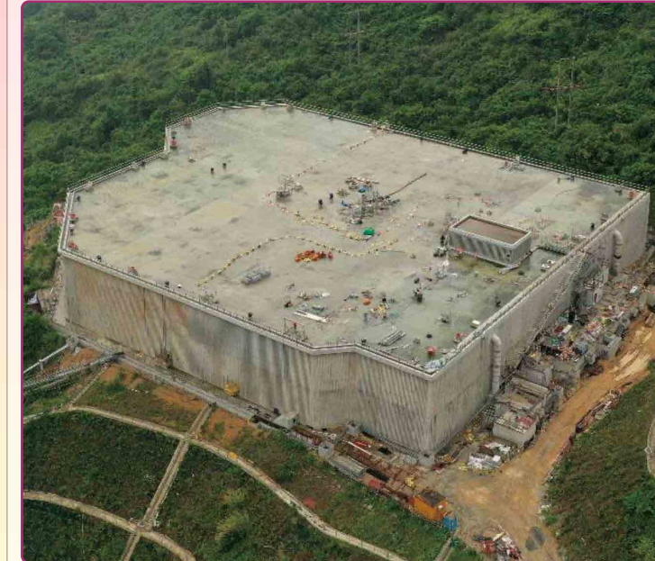
小蠔灣食水配水庫及相關鋪設水管工程已經大致完成 Siu Ho Wan Fresh Water Service Reservoir and Associated Mainlaying Works have been substantially completed
