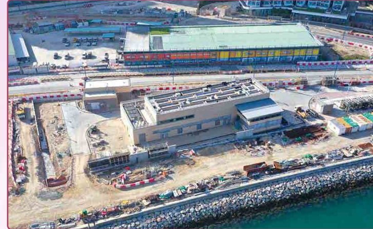
海水抽水站最後測試已經完成 Final stage of testing for Salt Water Pumping Station has been completed
