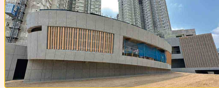
東涌河公園訪客中心的建築裝修及機電工程正在進行中 Architectural Builder's Work and Finishes (ABWF) works and Electrical and Mechanical (E&M) works for the Visitor Centre at Tung Chung River Park are in progress
