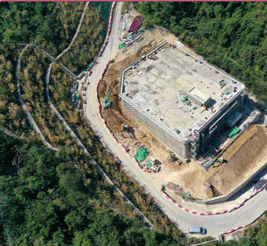
海水配水庫已在進行最後測試，餘下相關道路及渠務工程正在建造中 Salt Water Service Reservoir is currently in the final stages of testing. Related drainage and roadworks under construction.
