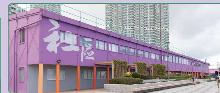
東涌社區聯絡中心是透過翻新及改裝舊有的駐地盤辦事處建造而成 CLC was constructed through renovation and modification of an unused site office.
