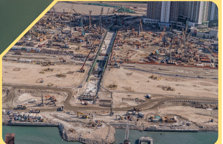
於新填海土地建造箱形排水暗渠 Construction of drainage box culvert on new reclaimed land
