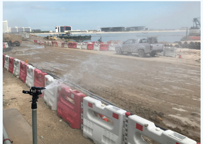
灑水器進行灑水 Spraying of water through sprinkler system
