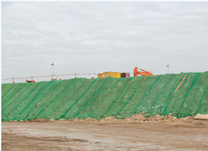
用防塵網覆蓋泥土暫存區 Covering the temporary stockpile by dust control mats
