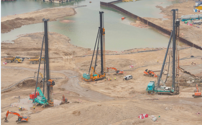
深層水泥拌合法機械 Plants for deep cement mixing works
