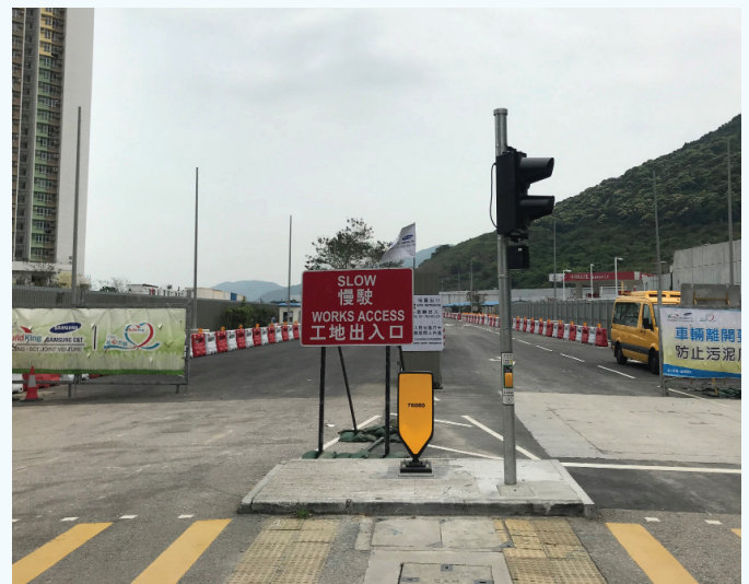
文東路、迎東路及迎禧路交界處的道路改善工程已完成 Completion of improvement works at the junction of Man Tung Road, Ying Tung Road and Ying Hei Road
