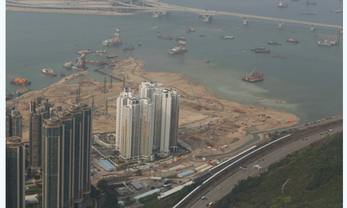
迎東邨對出的填海工程 Reclamation works outside Ying Tung Estate
