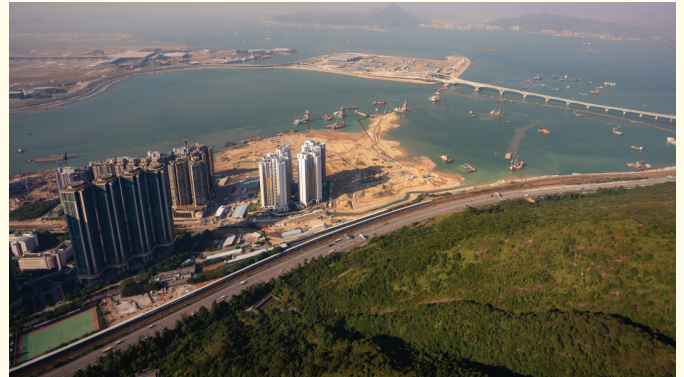
迎東邨對出的填海工程 Reclamation works outside Ying Tung Estate
