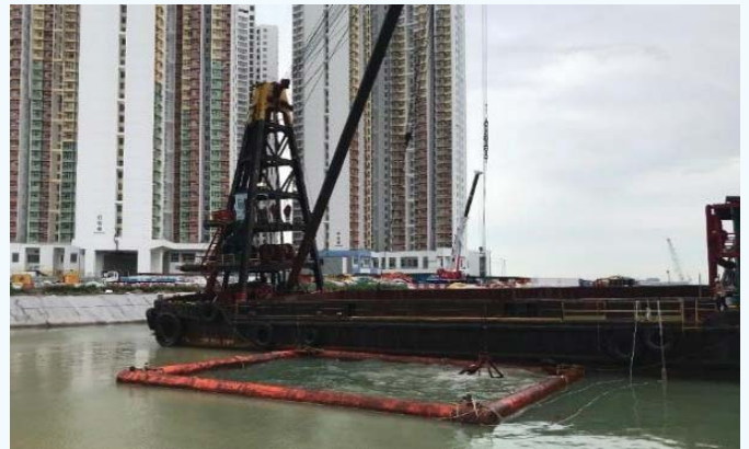
設置框架式隔泥幕 Setting up frame type silt curtain
