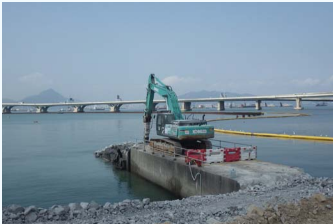
拆卸白芒碼頭 Demolishment of Pak Mong Pier
