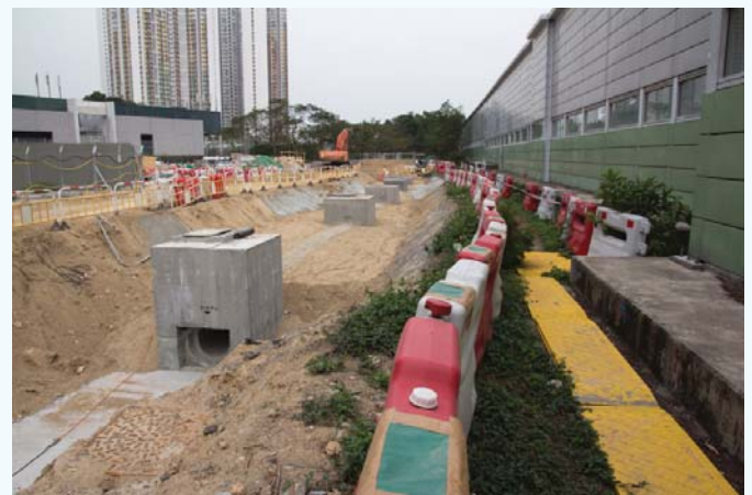
渠務工程(文東路) Drainage works (Man Tung Road)
