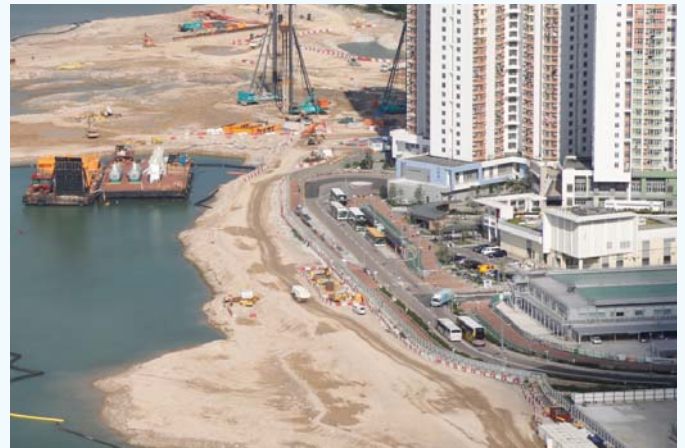
迎東邨對出的填海工程 Reclamation works outside Ying Tung Estate
