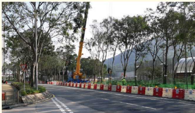
道路及渠務工程（文東路鄰近足球場） Roads and drainage works (Man Tung Road near football field)
