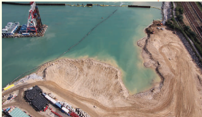
迎東邨對出的填海工程 Reclamation works outside Ying Tung Estate
