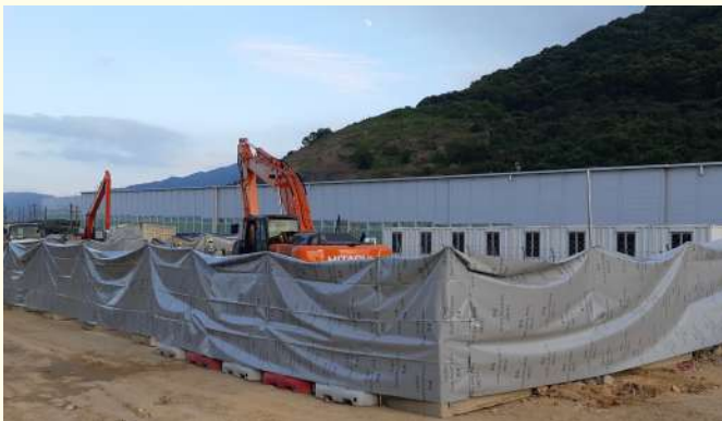
以屏障分隔工地 Setting up barriers during works
