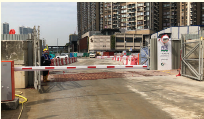
提供車輛閘門及交通指揮員以保障行人安全 Vehicular gates and traffic controller are provided to enhance pedestrian safety
