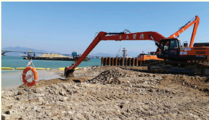
鋪設公眾填料 Placing of public fill
