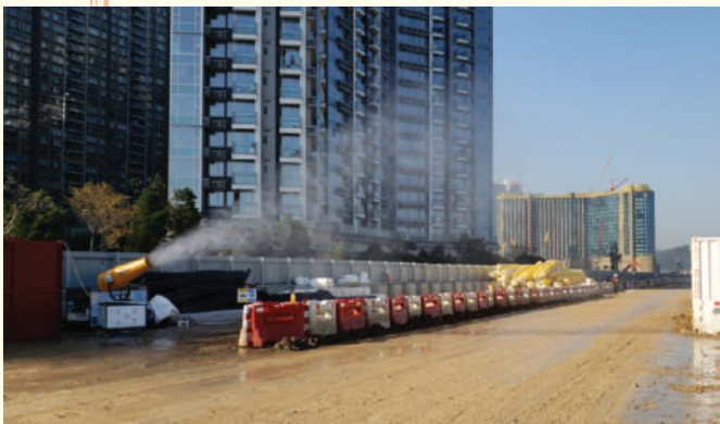
工地灑水 Water spraying at work site
