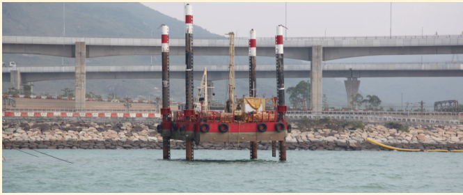
海上勘探 (進行中) Marine ground investigation (in progress)
