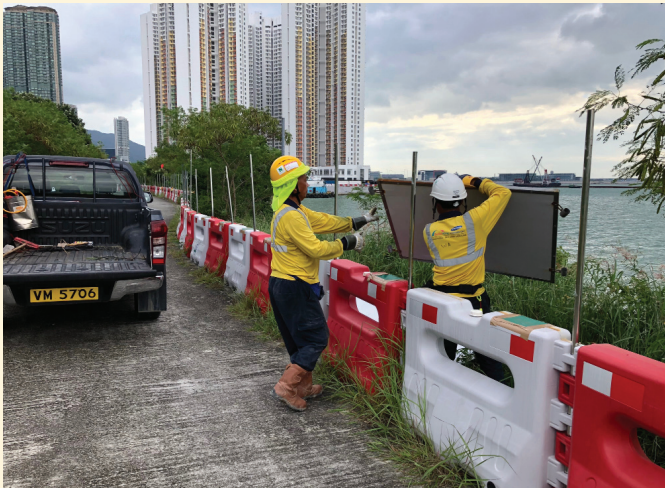
防風措施以免影響港鐵設施及公眾安全 Precautionary measures to avoid affecting the facilities of MTRC and public safety
