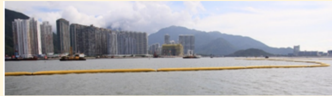
隔泥幕緩解工程對水質的影響 Silt curtain to mitigate impacts on water quality
