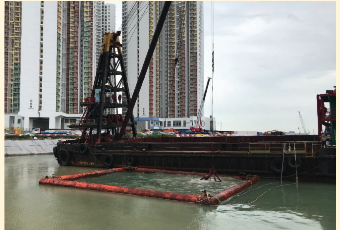
鋪設砂墊層(進行中) Placing of sand blanket (in progress)
